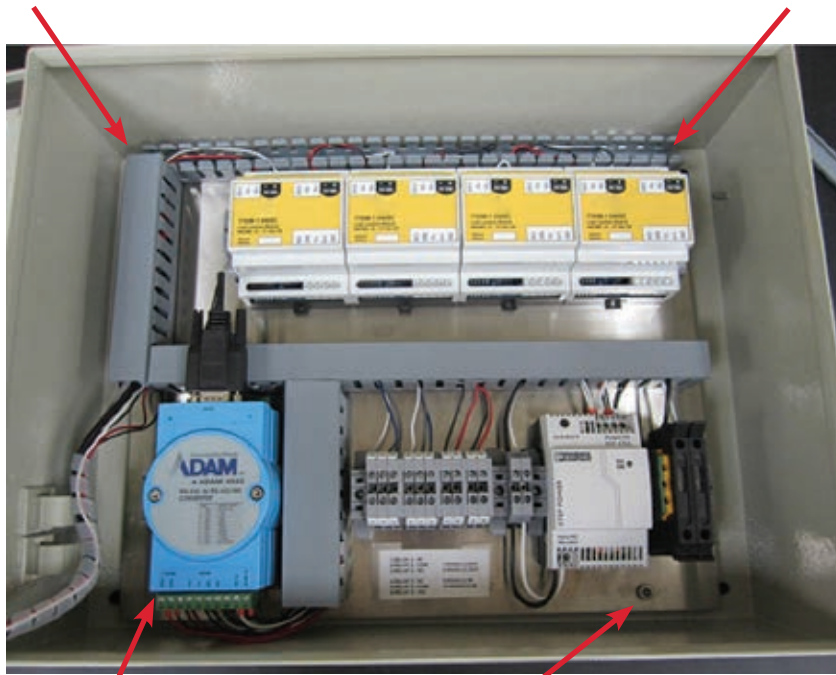
Back plane assembly securing bolt locations
